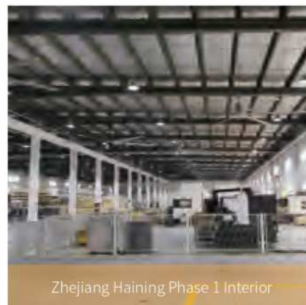
Zhejiang Haining Phase 1 Production Base
